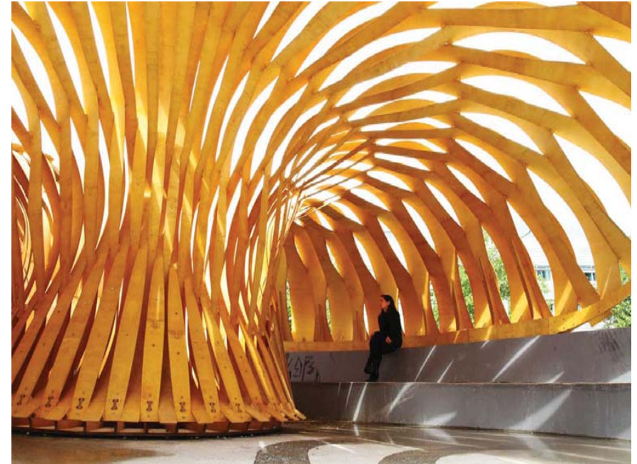
FIGURE 2_2: usage of bending-active structure. (Source: ICD/ITKE Research Pavilion 2010)
